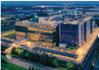
NTT-JKT3 Data Center Indonesia
