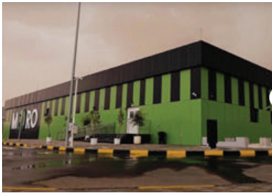
Moro Data Centre UAE
