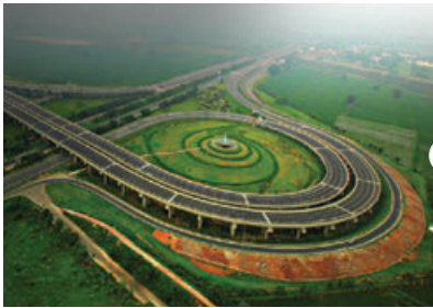
Yamuna Expressway India
